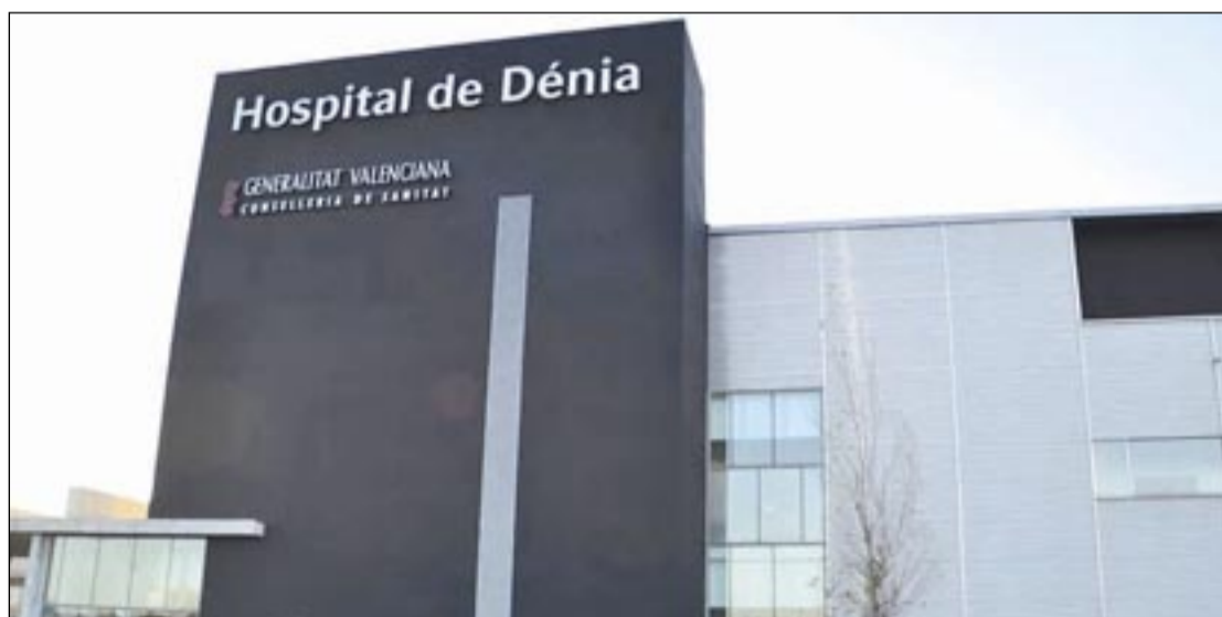
Vista general del hospital.
