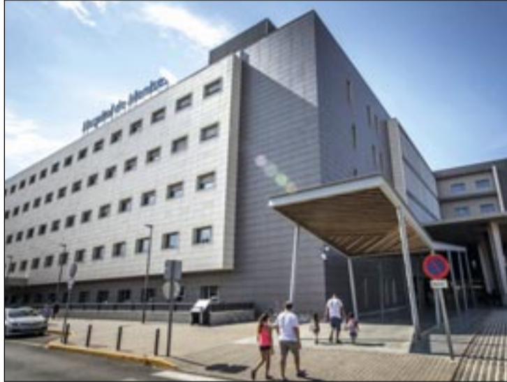
Vista general del hospital.
